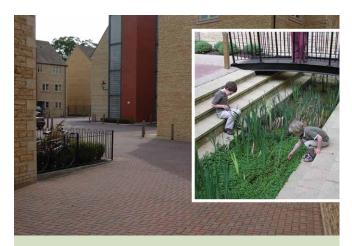
Water controlled and cleaned by extensive permeable paving feeds directly into a planted canal, then to a river.
