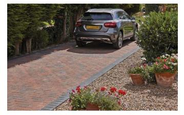
**Impermeable Surfaces** – such as conventional concrete block paving with sand joints, draining on-site to:
