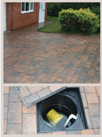
Around this home, rainwater runoff collected from all impermeable surfaces including roofs and paths, together with the 60m<sup>2</sup> permeable drive itself, passes into the tanked permeable pavement which contains a concealed sump. Here, a small pump is used to draw off the harvested water, in this case for outside uses, via a tap and hosepipe.
