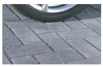
Permeable paving should have permeable aggregate filling the joints
