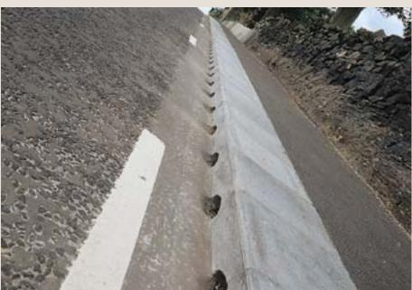
Precast concrete kerbs systems are available with integral drainage facilities
