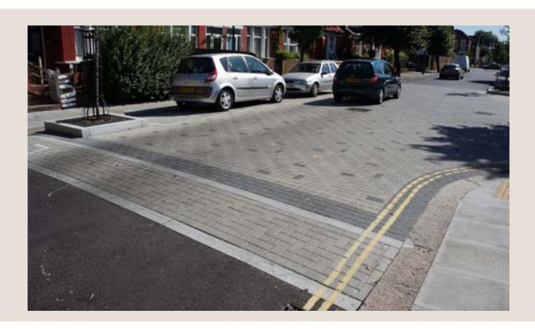
Precast concrete paving meets all these requirements and MfS highlights its own research demonstrating that block paving significantly reduces traffic speed compared with asphalt, particularly on shared surfaces. MfS2 also identifies a number of key characteristics, identified in ongoing research of shared spaces, where precast concrete paving can play an essential role, including:
